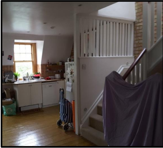
Open plan kitchen to means of escape stairs.
